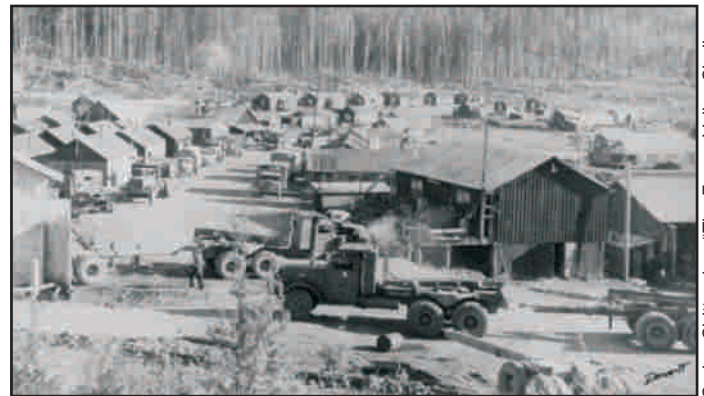
One of several Decco-Walton logging camps in the Skagit – this one near International Point Day Use on Ross Lake.
